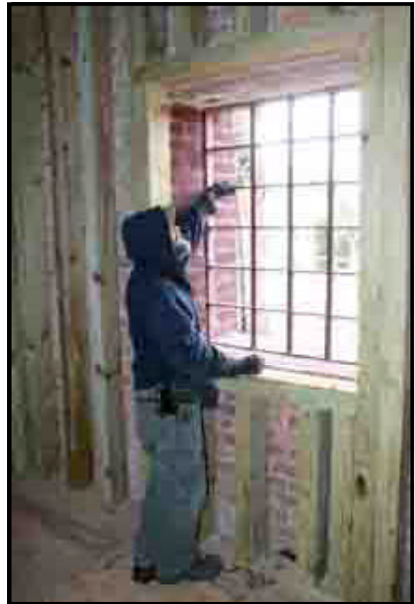
Fritz installing the iron bars in the first window.
