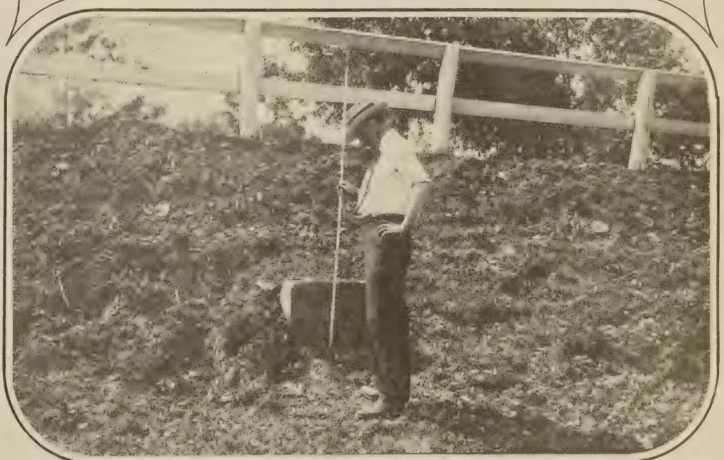
TOP - WATER AT BOTTOM OF 8-INCH SURFACE TREATED MACADAM ON A 6-FOOT FILL.
