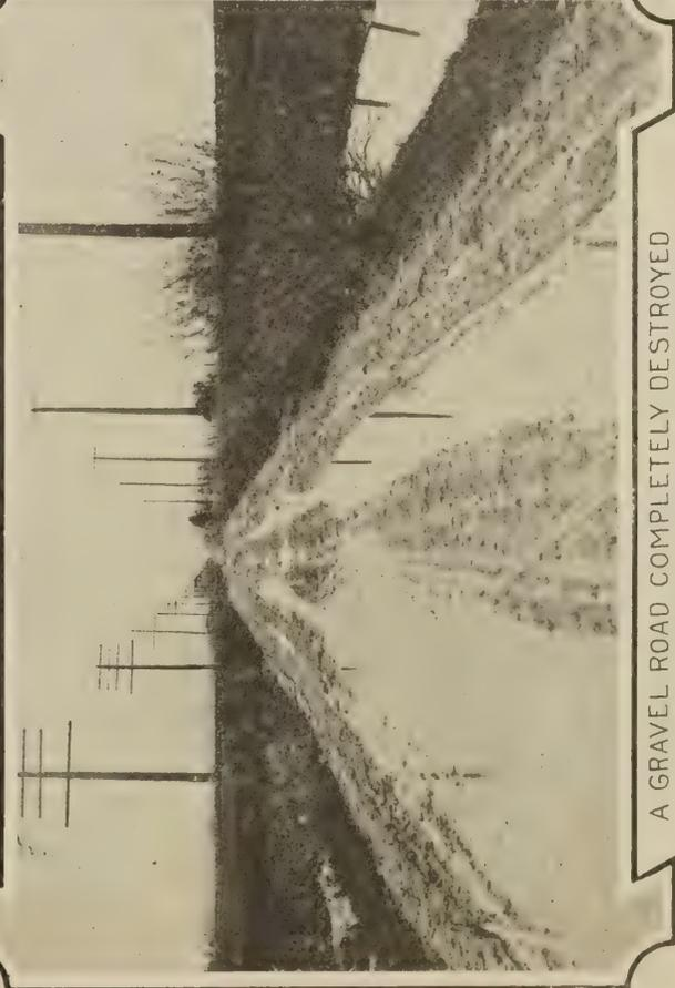
A GRAVEL ROAD COMPLETELY DESTROYED ON ACCOUNT OF POOR DRAINAGE.
