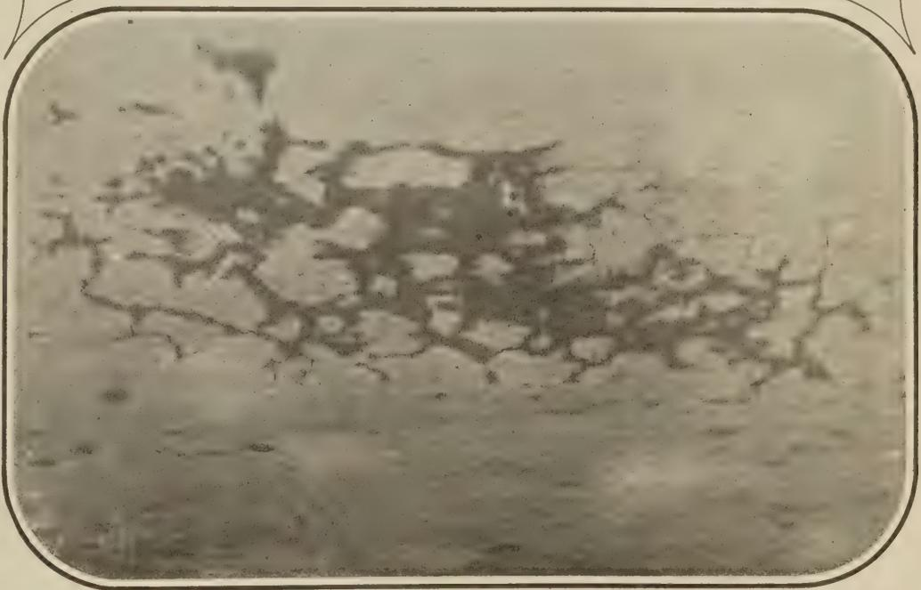
TOP - WATER STANDING IN MUD HOLE ON SHOULDER AT EDGE OF PAVEMENT ON 5-FOOT FILL. BOTTOM - MOISTURE BEING SHOVED THROUGH FROM BASE OPPOSITE MUD HOLE SHOWN AT TOP.
