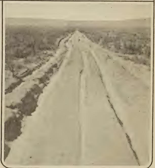
AT TOP—NATURAL SOIL ROAD IN NEVADA, WHICH BECAUSE OF THE EXCELLENT GRAVELLY SOIL IN WHICH IT IS LOCATED REQUIRES BUT LITTLE MAINTENANCE
