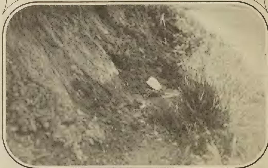
TOP-FAILURE IN 6-INCH CONCRETE ROAD DUE TO SOFTENING OF SUBGRADE BY WATER BEING ABSORBED FROM DITCH WHICH HAS BEEN FILLED UP AND NOT CLEANED OUT.
