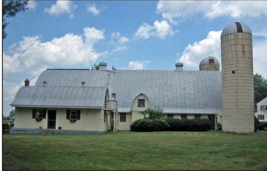
FIGURE 24: Gothic Arch Barn and Milk House, Atoka Forge Farm, near Atoka
