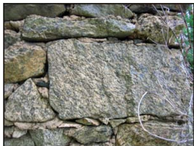
FIGURE 2: Detail of Stonework on a Fauquier County Building
