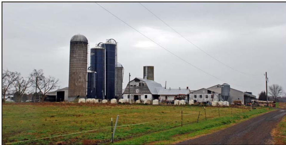
FIGURE 30: View of Dairy Farm with Concrete Stave Silos and Harvestone Silos near Elk Run
