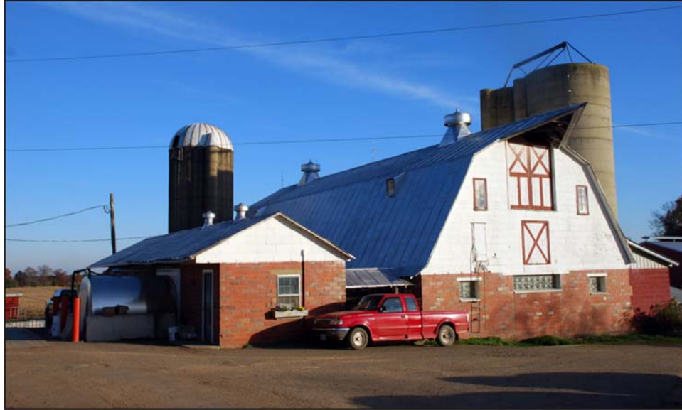
FIGURE 20: View of Dairy Barn and Milk House Featuring Structural Clay-Tile Construction, near Midland
