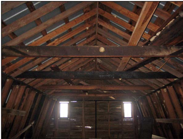
FIGURE 21: Interior of Dairy Barn Framing
