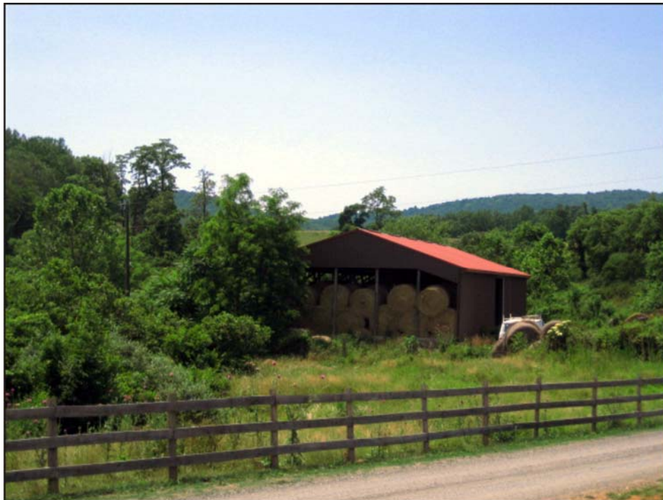
FIGURE 35: View of Pole Barn near Markham Used as a Hay Barn
