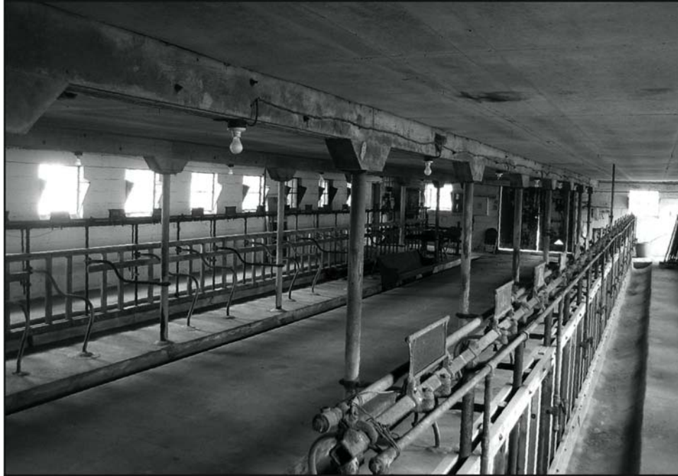
FIGURE 19: Interior of Dairy Barn Depicting Concrete Floors and Gutters
