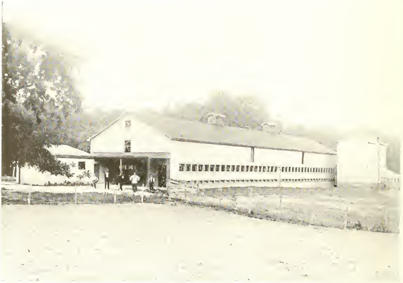
Sanitary Barn and Silo near Richmond, Henrico County.
